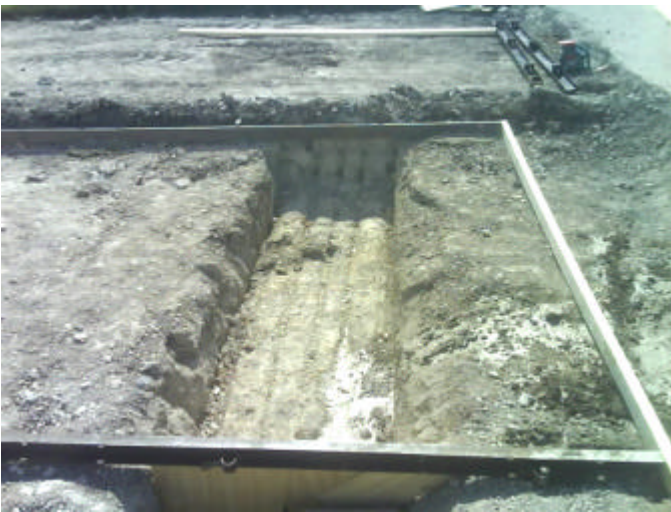
Deeper trenches where load cells will sit on the concrete
